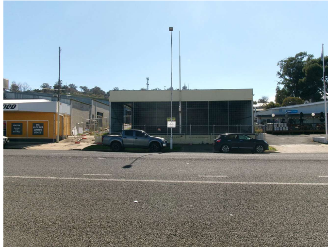
Figure 3. Kendal Street Frontage
