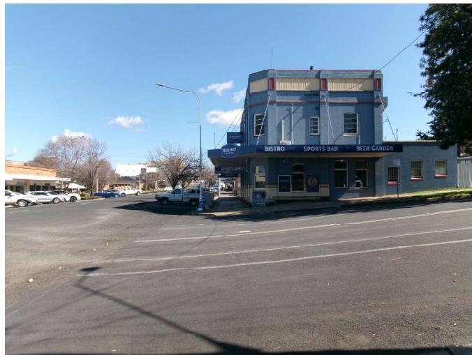
Figure 6. 154 Kendal Street, Railway Hotel
