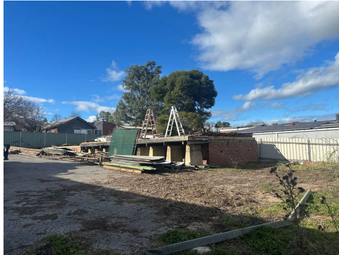
Figure 5. Partial Demolition of Existing Shed (Approved DA no 10.2025.36.1)
