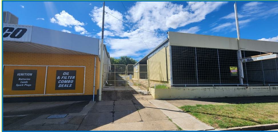
Figure 3b Photograph of the Site Frontage from Fitzroy Street (driveway)
