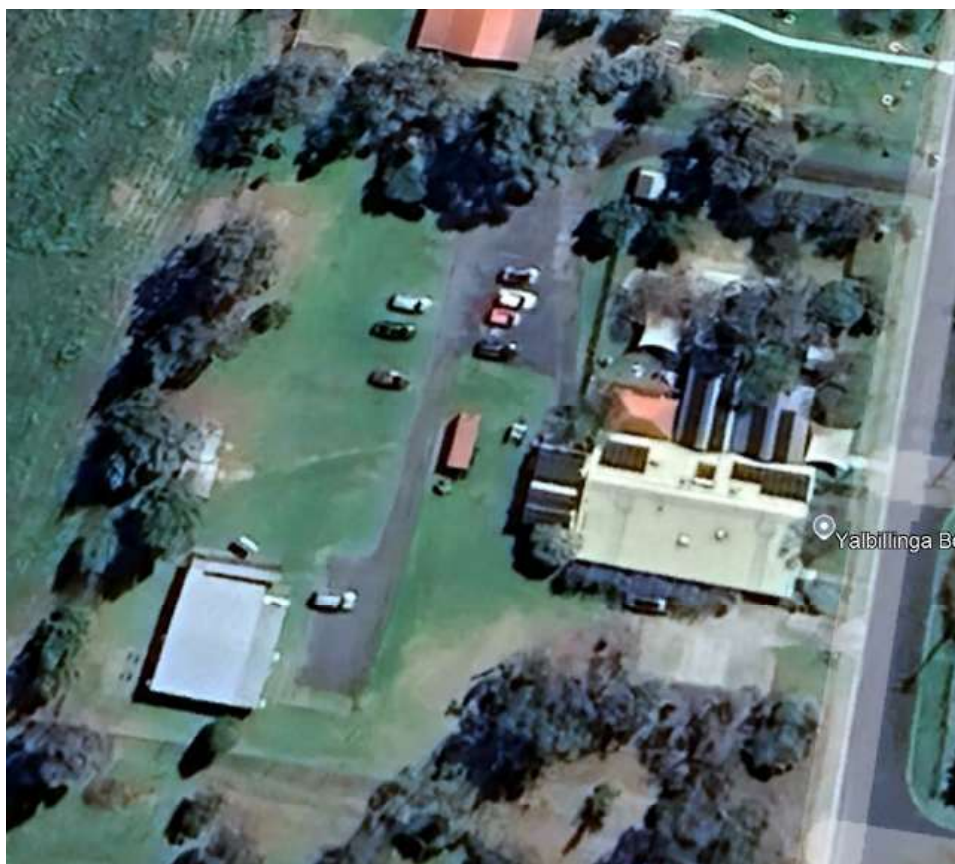
Image 2: Existing informal staff parking arrangement onsite. Source: Google, accessed 29/05/25.
