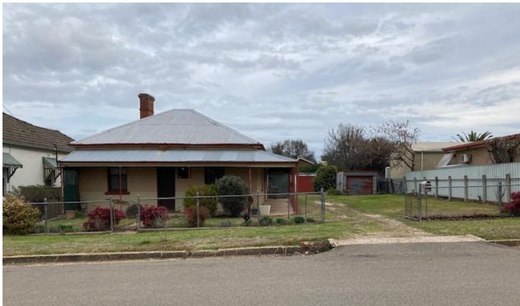
3 Railway Street - existing street view.
