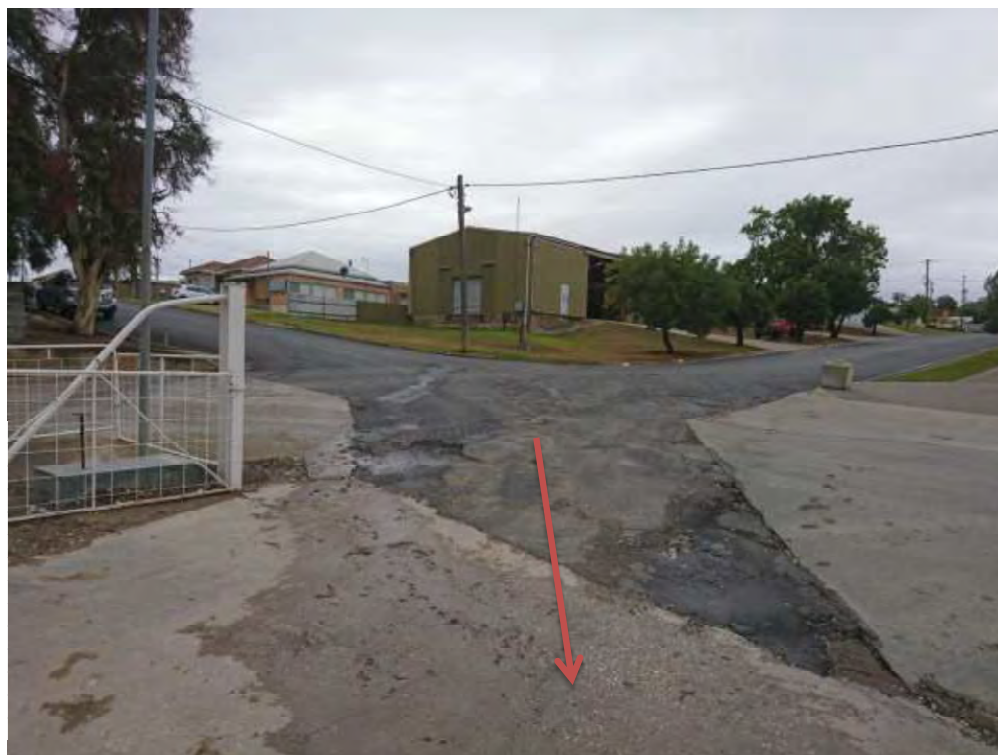
Figure 3 – Significant run-on occurs from the street junction onto the Project Site entrance
